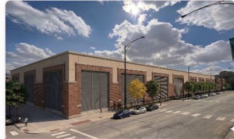
THE PROPOSED SUBSTATION
